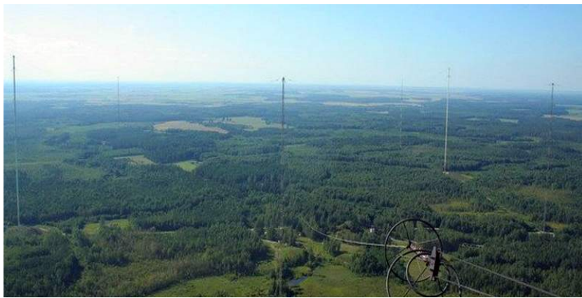
FIG. 1: Long-range submarine communication centre “Vilejka” of the USSR Navy. The height of antennas: 305 m. Radiated power: 1 MW. Distance: 10 000 km, water penetration depth: 60-70 m.
